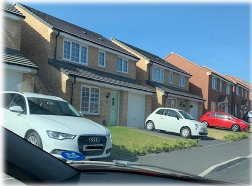
Figure 21: View of integral garages in the development
