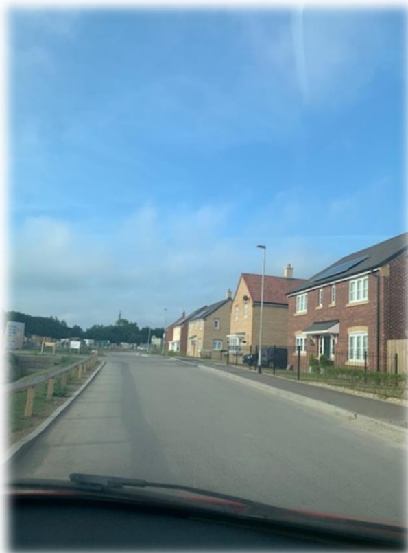
Figure 11: View along the development from Swinderby Road
