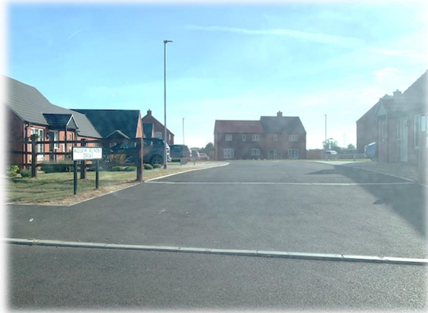
Figure 12: View into the site from the entrance
